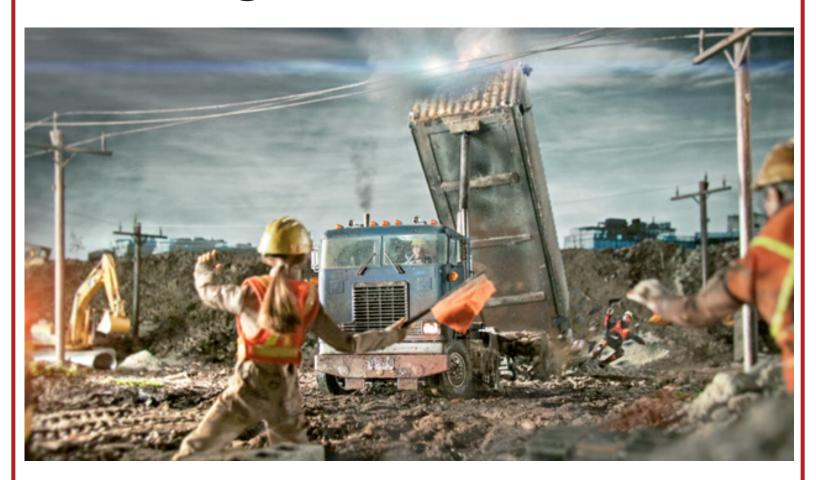
While working near overhead power lines it is always important to know your surroundings. It is important to remember that the vertical clearance to overhead power lines ranges from 10-12 feet depending on the voltage.
